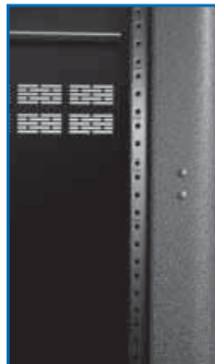
Hash marks on rails indicate rack unit increments
